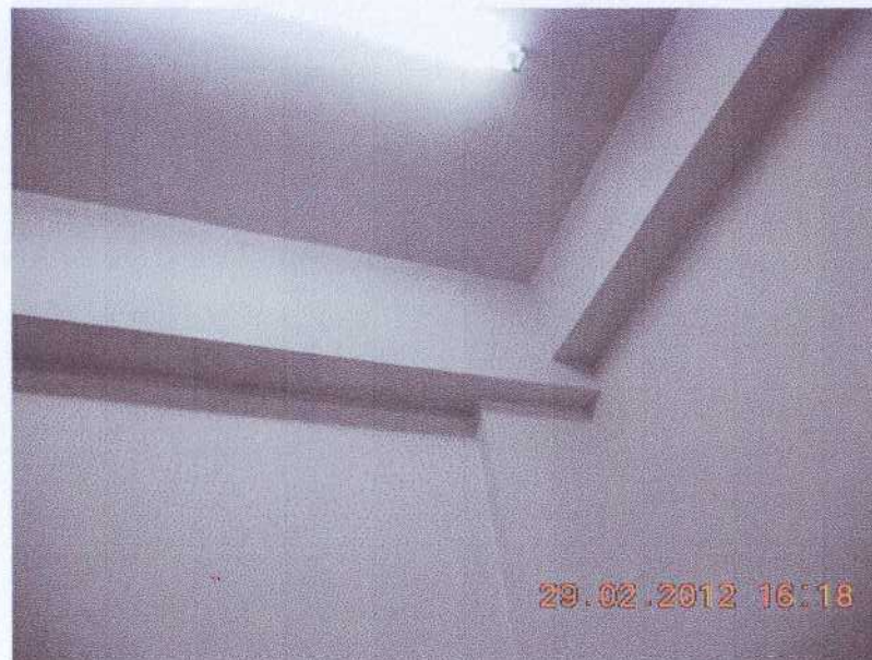
Extruded concrete removed and repaired
