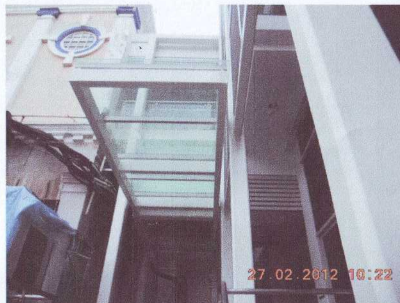
un even welding smooth& repaint completed
