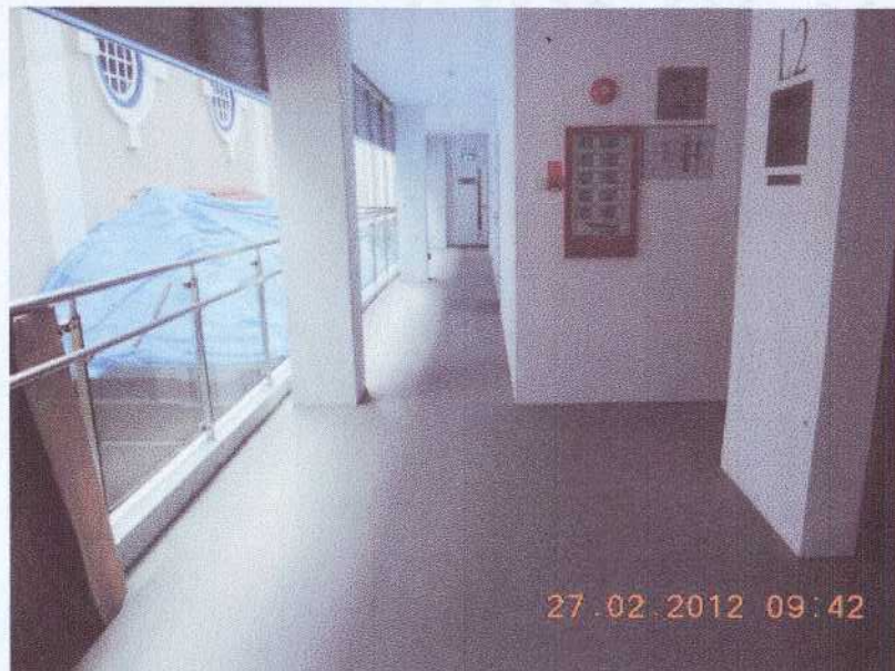
Self leveling screed was completed all corridors and staircases
