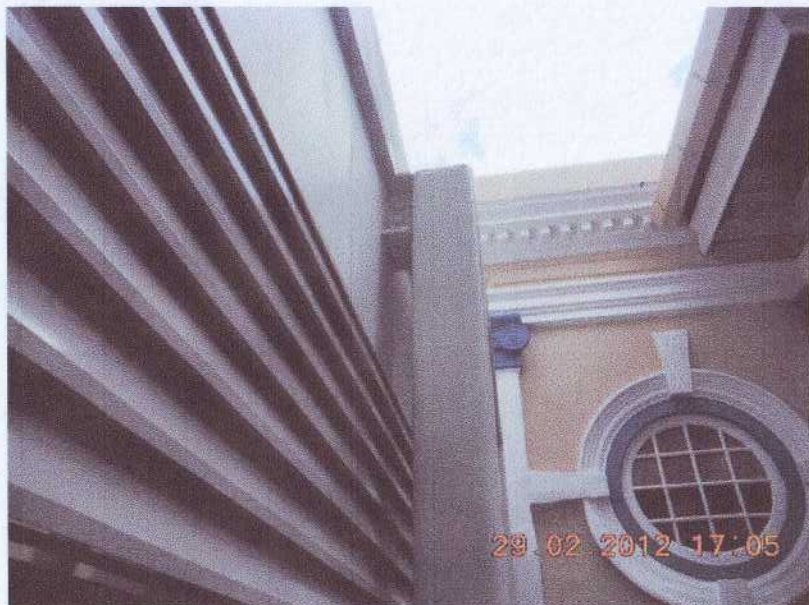
Vermiculite paint removed from I beam
