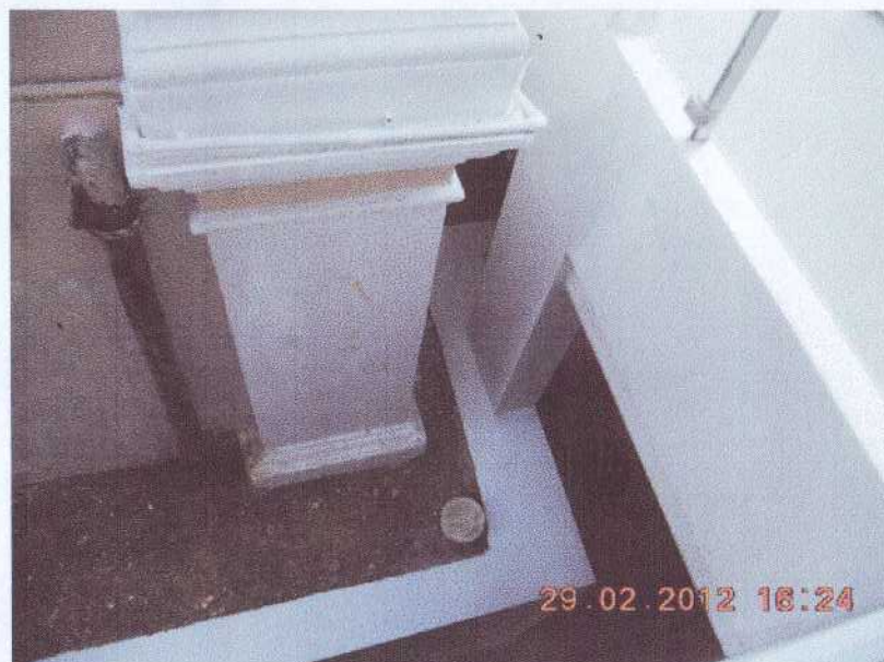
Protruded I beam&steel plate removed
