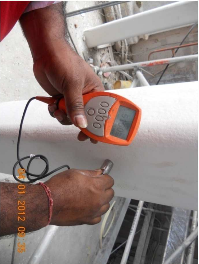
Intumescent test completed on 4 column
