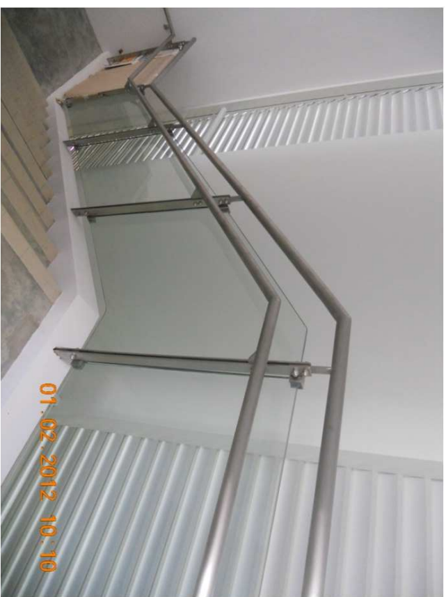
St -02 completed with handrail & glass
