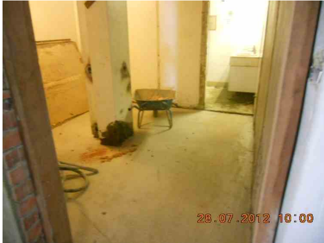
Visitor centre slab construction completed at 1 st STY.
