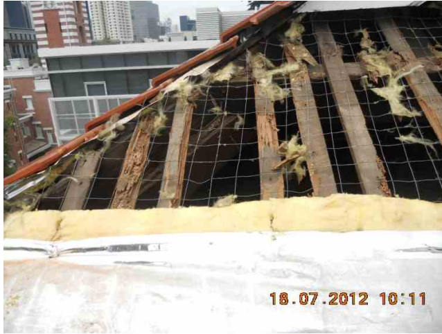
Removing of timber battens and relaying of clay tiles in progress.
