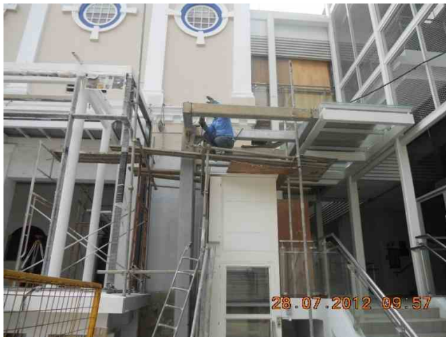
Erection of steel members completed at platform lift canopy
