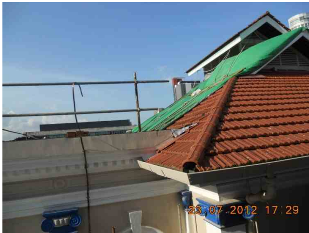
Protection during changing of clay tiles
