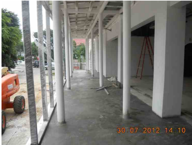
Roof completed at right wing
