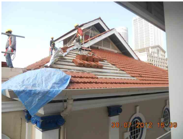
Relaying of clay tiles in progress at pitch roof.
