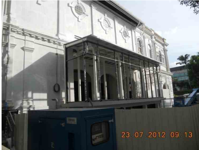
Left wing completed with roof and gutter
