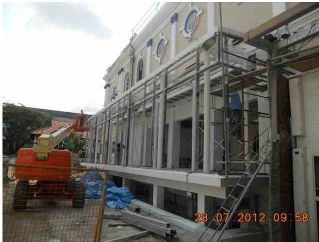
Right wing in progress with installation of gutter & roof.
