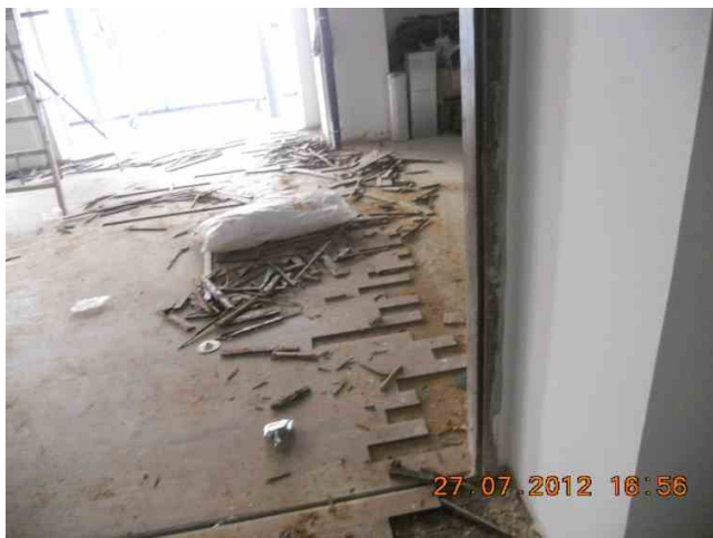
Repairing of timber flooring in progress at 1 st STY
