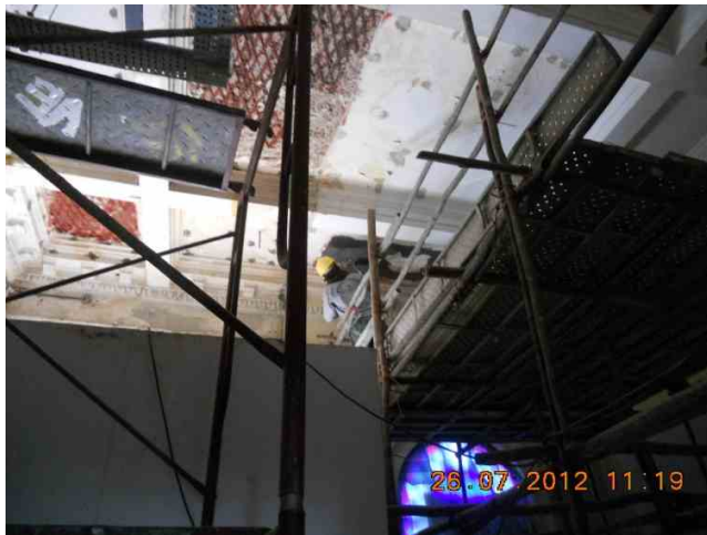
Repairing of roof slab soffit in progress at 2 nd STY
