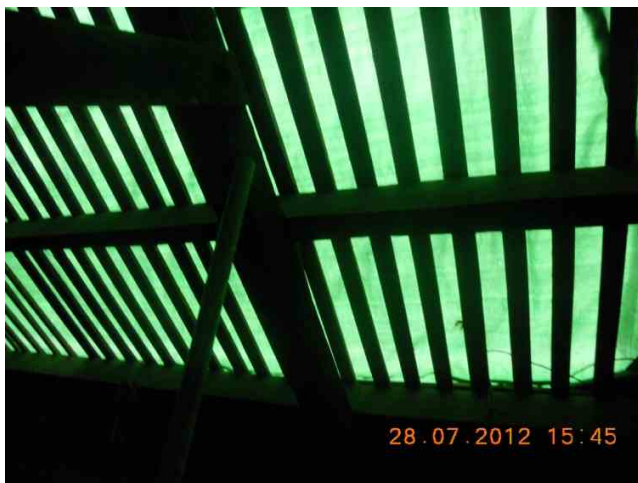
Replacing with new timber battens in progress at pitch roof.
