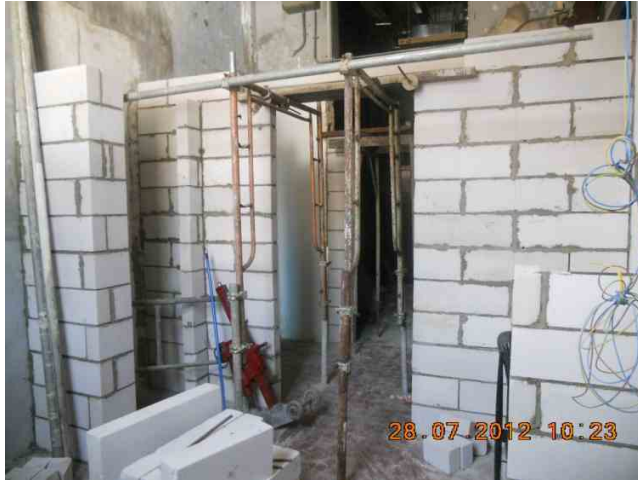
Erection of light weight concrete wall at new changing room
