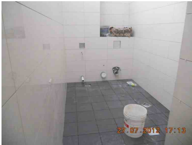
Tiling works completed at 1 st STY toilet
