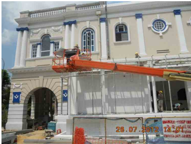
Painting in progress at right side of conserved building
