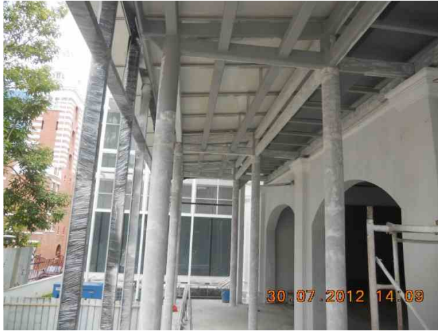
Smoothing of beams and column in progress at left wing
