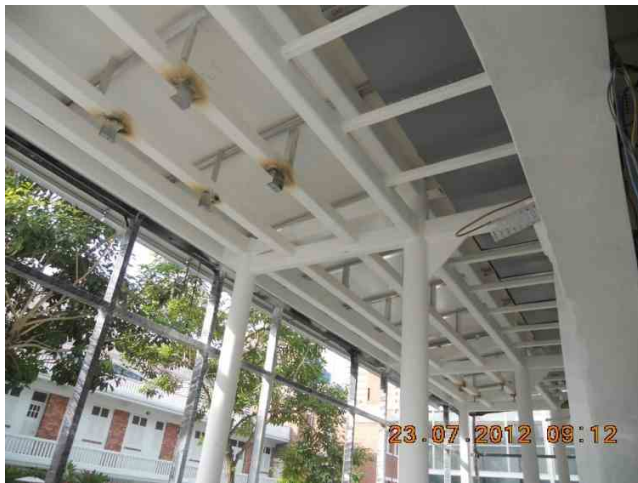
2 hr fire rated intumescent paint completed at both side wings
