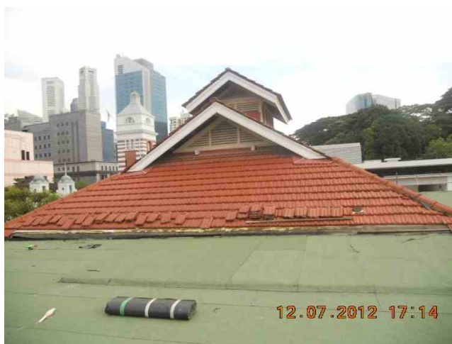
Laying of water proof membranes completed.
