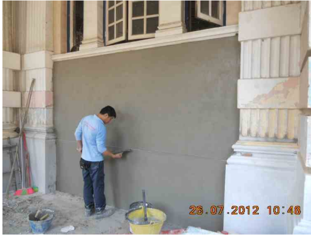
Re-plastering in progress at car poach
