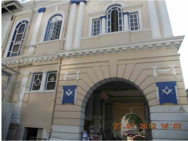
Painting in progress at left side of conserved building.
