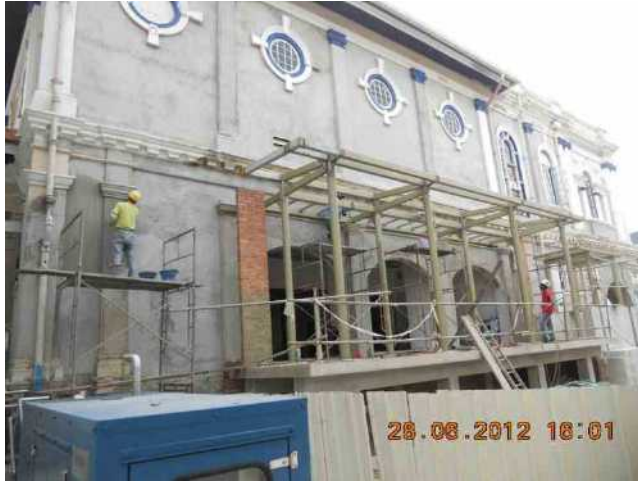
Re-plastering of side facades completed with final coat. Both side wings steel structure completed.
