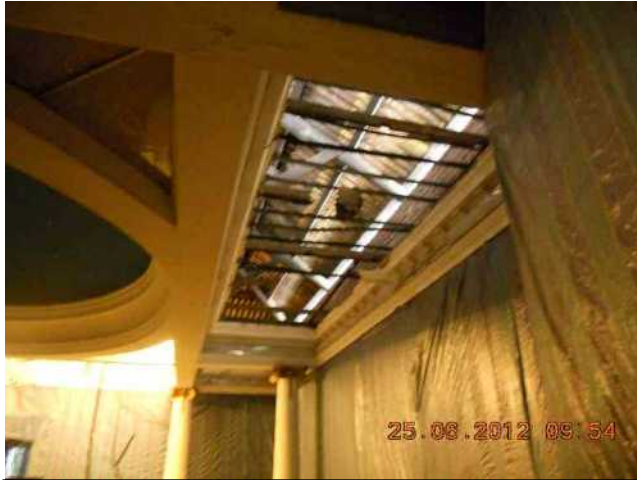
Existing ceiling completely removing from main temple room.
