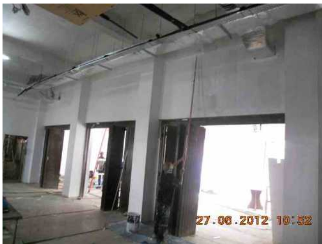
Painting, ACMV, Electrical and plumbing in progress at 1 st Storey
