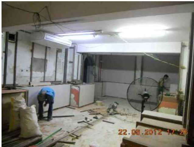
Erection of Ventilated wall in progress at basement.
