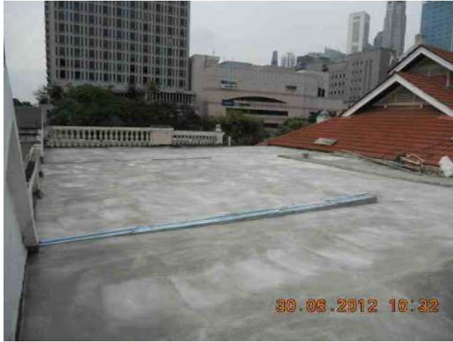
50mm thick granite chipping casting completed with insulation board.
