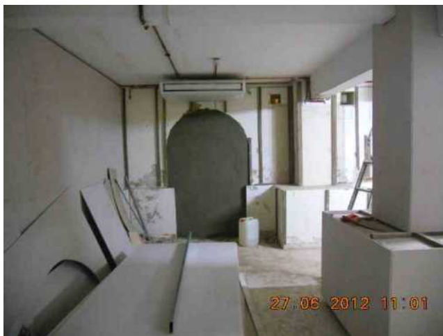
Partially completed ventilated wall with opening closed to form a celler.
