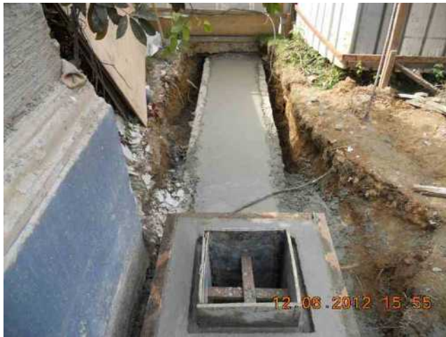
Drain connection to main completed on both side.
