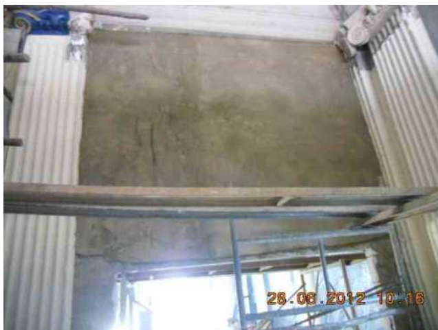
Light weight wall completed at 2 nd STY stair lobby.
