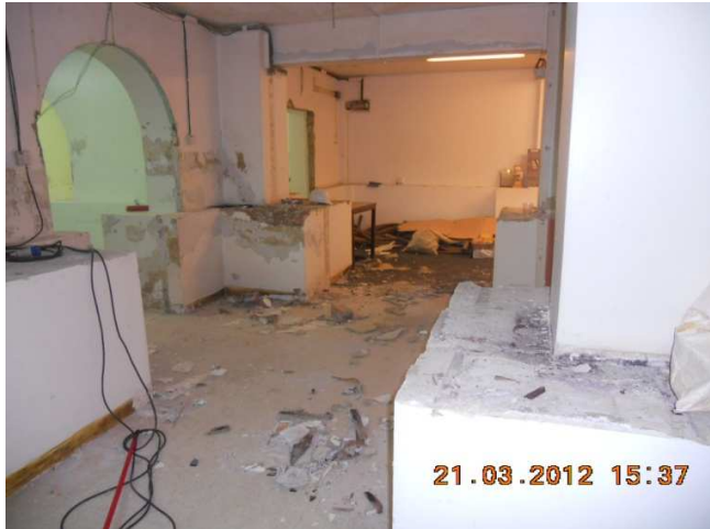
Removing of existing paint & loose plaster @basement
