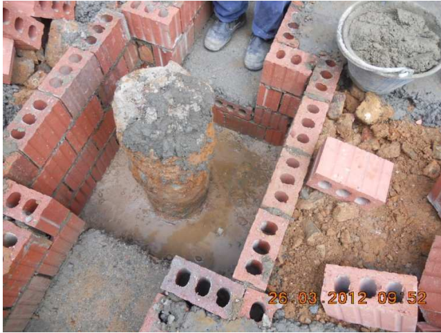
Lean concreted at micropile cap at right wing
