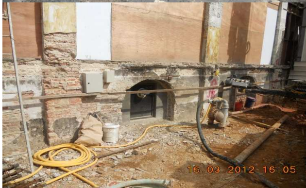
Vibration-meter & settlement marker installed before piling
