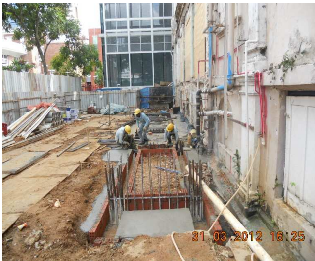
ST-06 footing completed & ground floor is in progress
