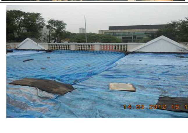
Protection on the roof (cover with canvas)
