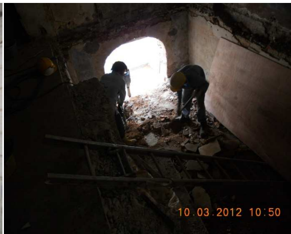
ST-04 breaking slab and footing completed
