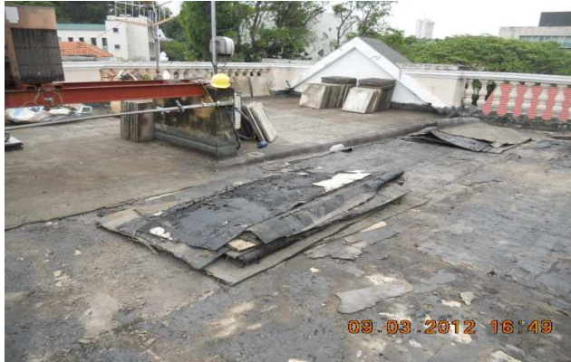
Removing of existing membrane completed
