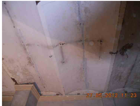
Clean the crack & prepare for Epoxy injection at the 2 nd STY slab soffit.
