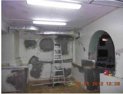
ACMV work start on the 28 th of May
