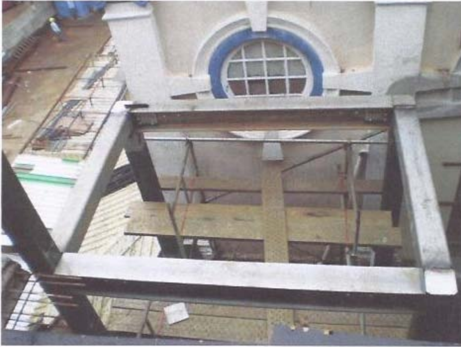
Erection of steel beams to roof of Link Bridge in progress.
