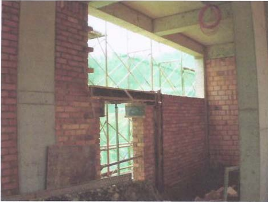
Laying of brick walls at 3 rd storey in progress.
