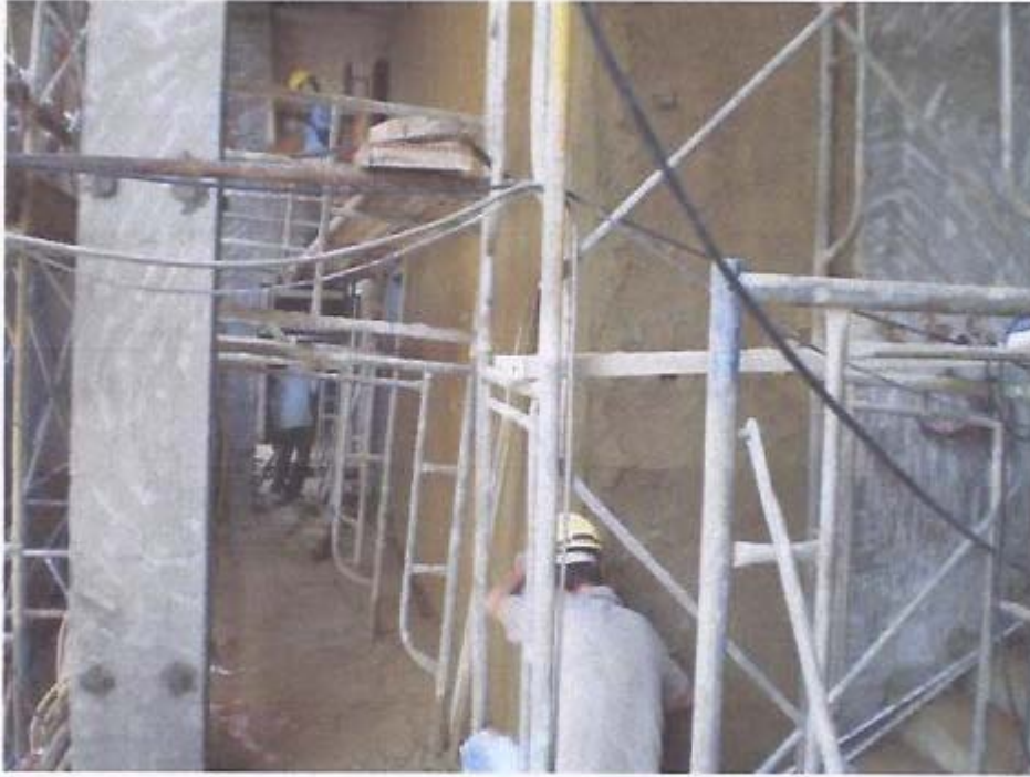
Plastering to 1 st storey brick walls in progress.
