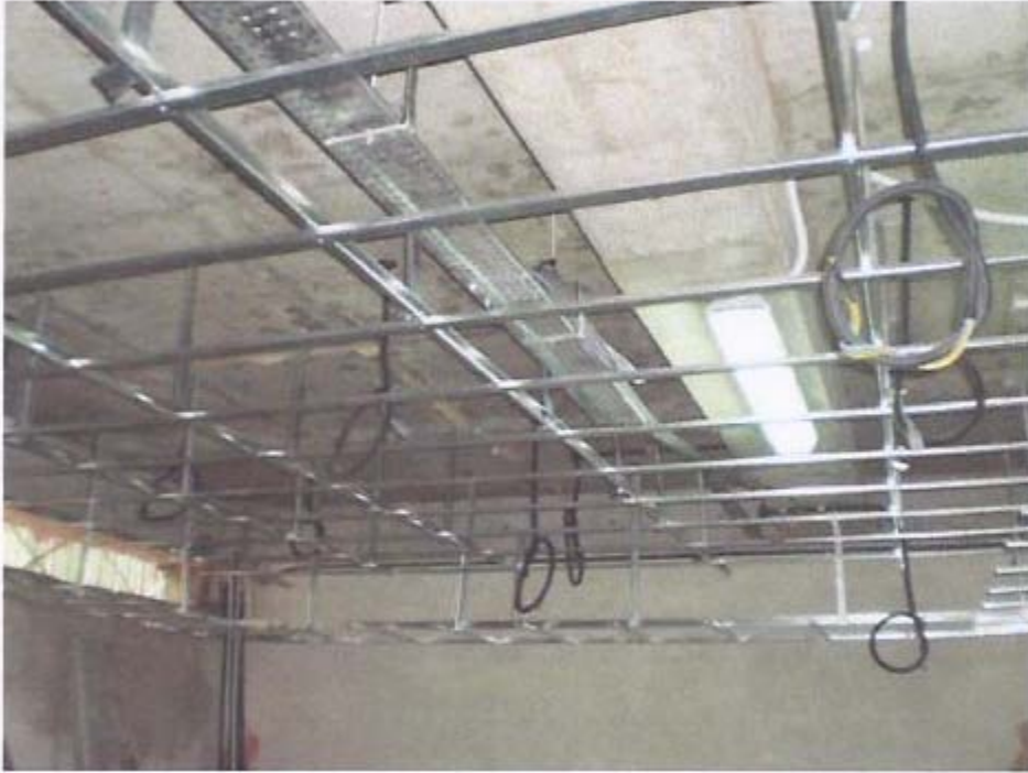
Installation of ceiling to basement in progress.
