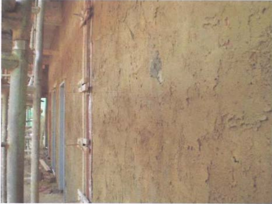
Base coat of cement / sand plastering to 3 rd storey completed.
